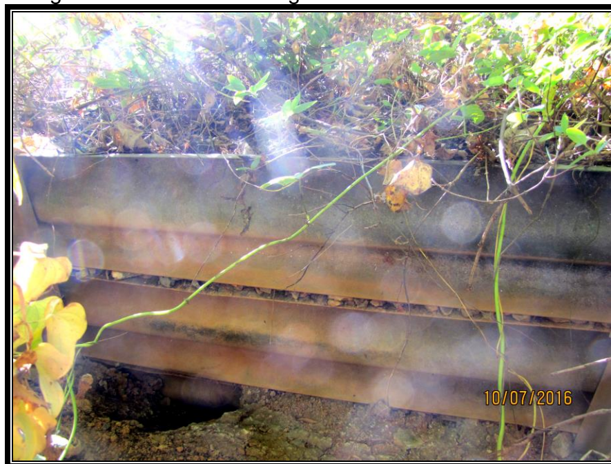
Figure 2 Site 1 - Guardrail retaining wall to be removed.
